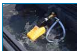
Float valve equipped with an anti-splash housing.
