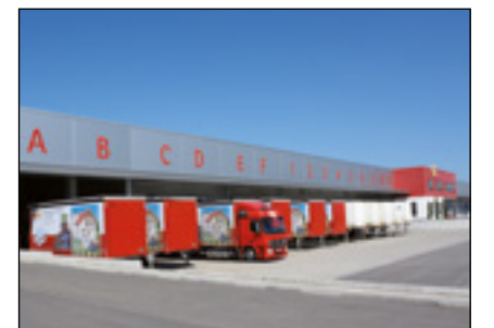
Teningen logistics centre
